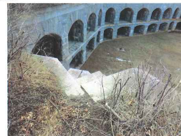
INSTALL STEEL GUARD RAIL ALONG STAIRWAY. SEE SHEET C-506 FOR DETAILS. REFER TO PHOTO 4 ON THIS SHEET. INSTALL STEEL BARRICADE RAIL AND GATE AT PORTIONS OF TOP OF STAIRWAY. SEE DETAILS B1, B4, AND B7 ON SHEET C-505. REFER TO PHOTO 1, 2, & 3 ON THIS SHEET. LOCATION OF GRANITE STAIRWAY SHOWN IS IN AN APPROXIMATE MANNER ONLY. REFER TO NOTE 9 ON SHEET G-101. PHOTO 1 PHOTO 2 PHOTO 3 PHOTO 4 PHOTO 5 GRANITE BLOCK TOP OF GRANITE BLOCK WALL STAIRS 6' WIDTH
