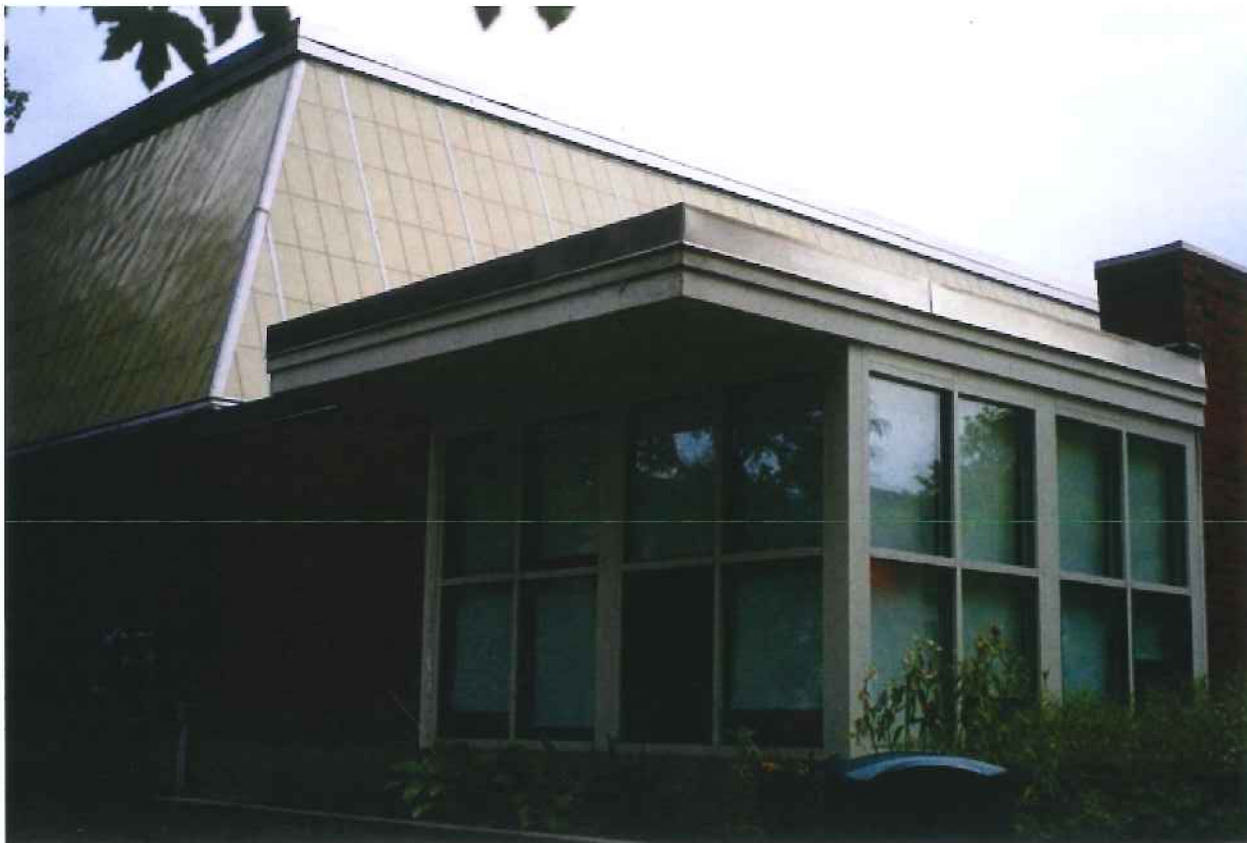
H - Existing Gym
