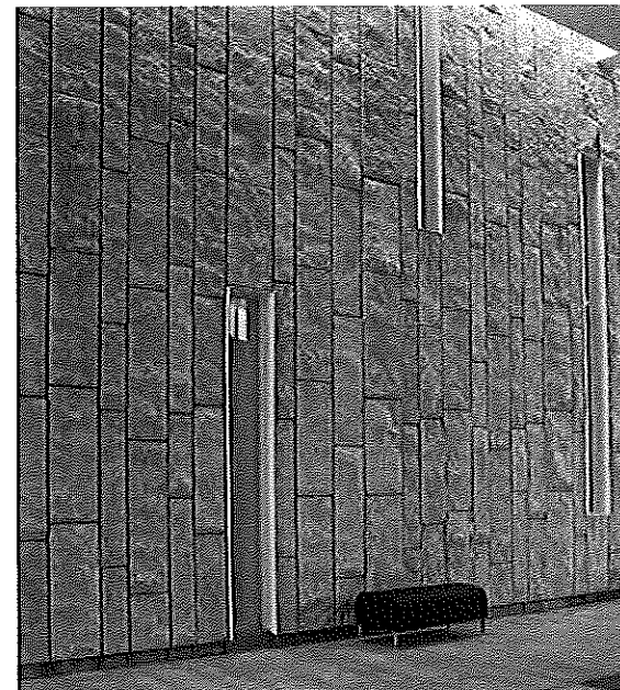
24" x 48" Arriscraft Adair Limestone Medium Dressed, Fleuri Anchored Dimensional Stone Vertical Running Bond Installation
