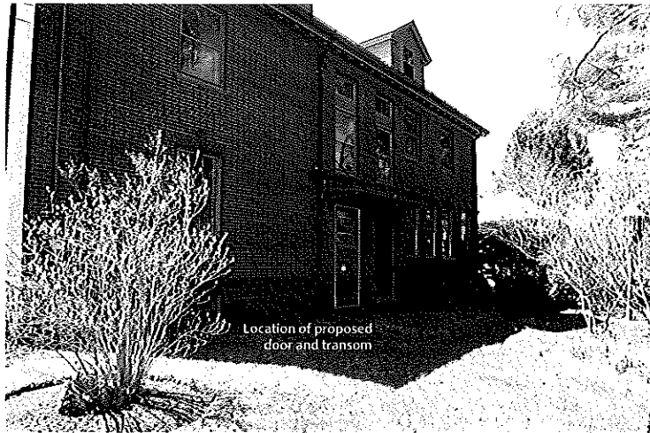
View of North Elevation
