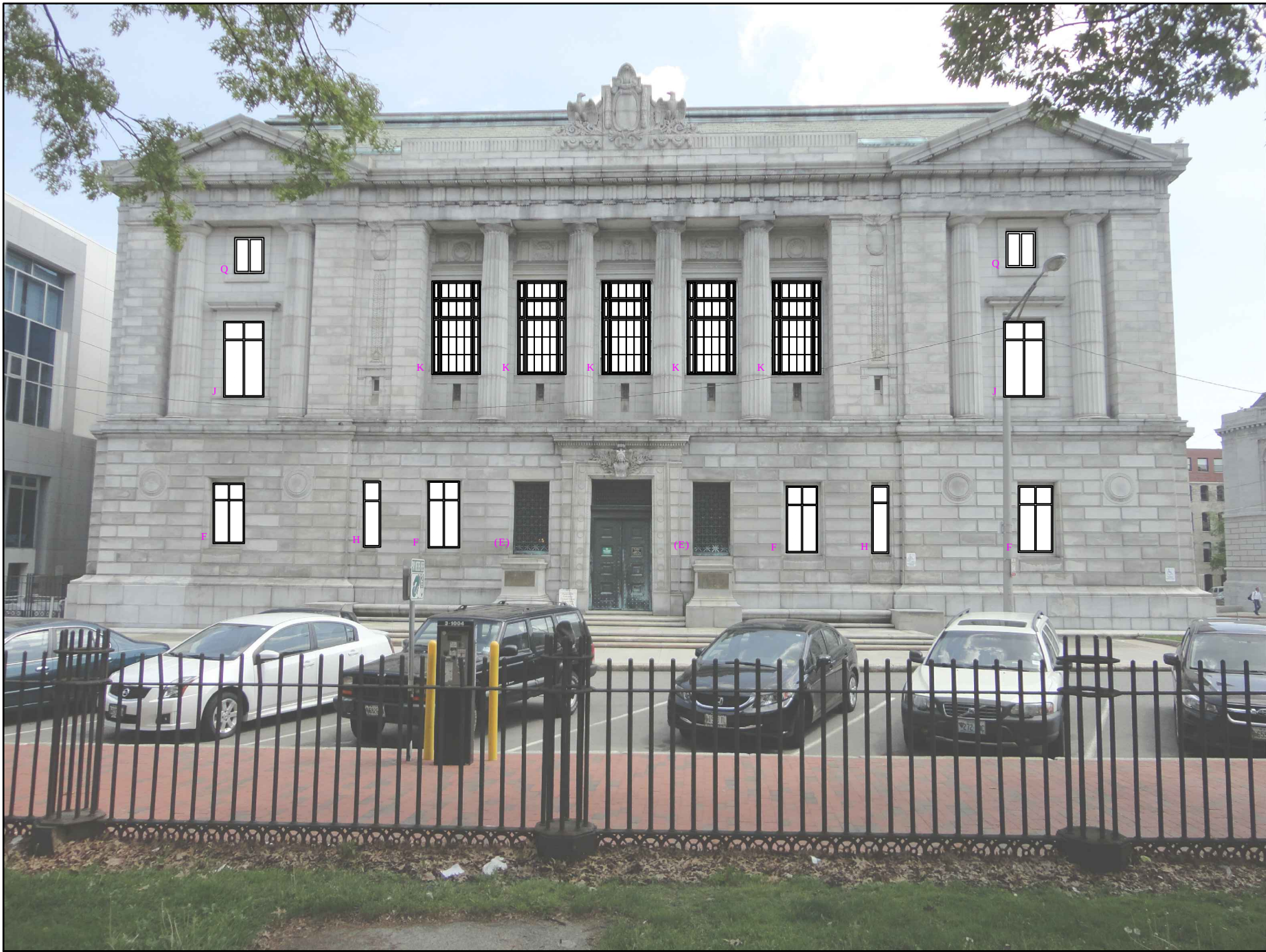
FEDERAL STREET FACADE
