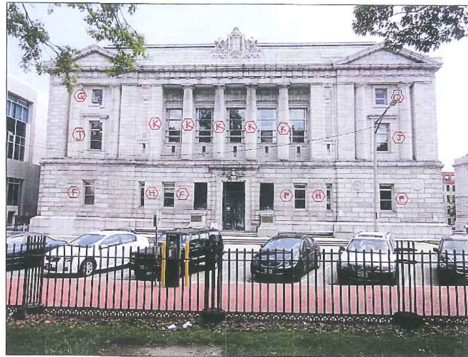
FEDERAL STREET FACADE
