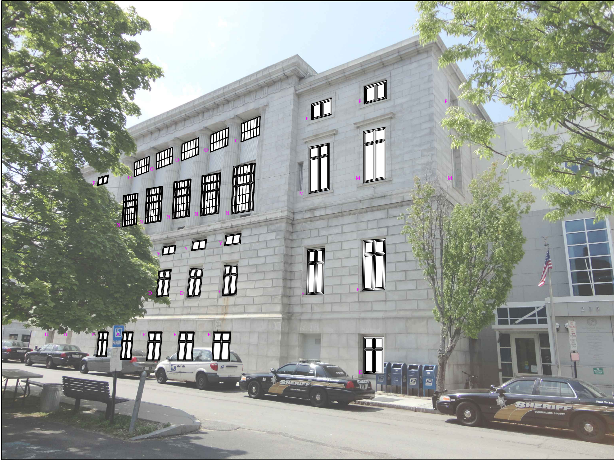
NEWBURY STREET @ CONNECTION TO NEW ADDITION
