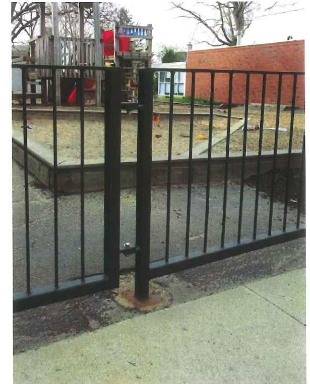
Powder Coated Steel Fence
