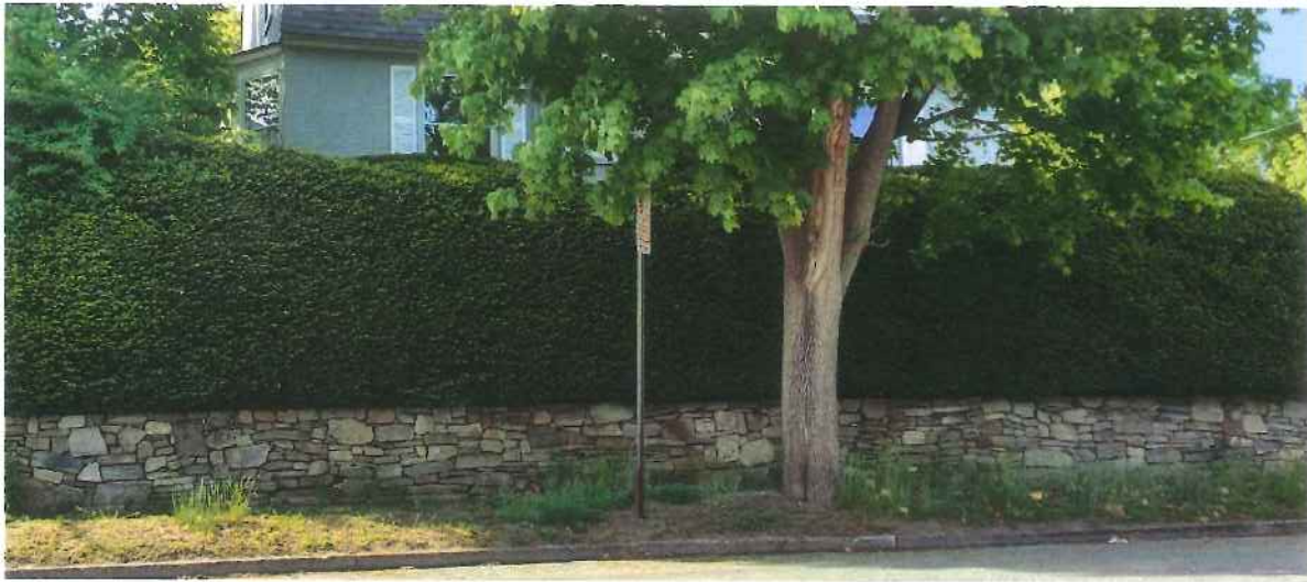
361 Danforth Street - wall height >30" with very tall hedge behind
