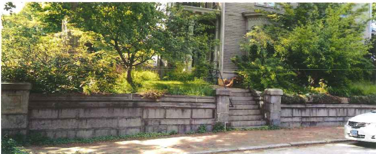
384 Spring Street – wall height +/-48" down to +/-28"
