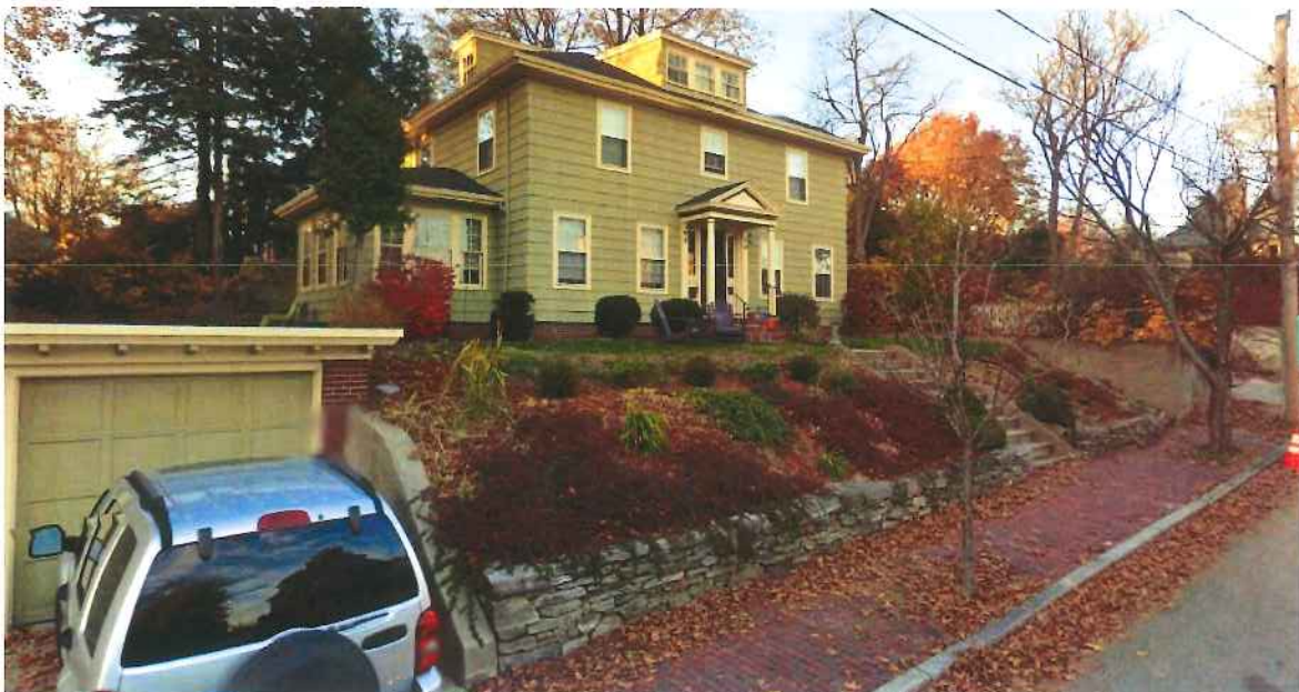
21 Orchard Street – wall height ranges from +/-28" (left side) to +/-16" (right side)
