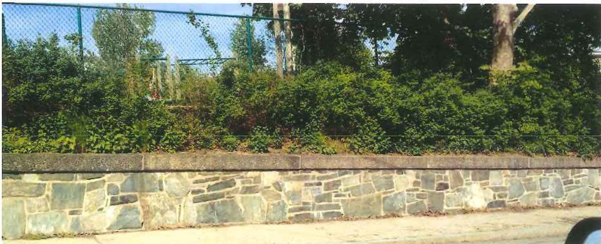
Waynflete School (Fletcher Street) - wall height >30", slope up played, heavily planted with tall vegetation, and large chain link fence
