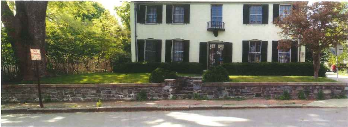
5 Orchard Street – wall height ranges from +/-36" (left side) to +/-40" (at steps) to +/-28" (right side)
