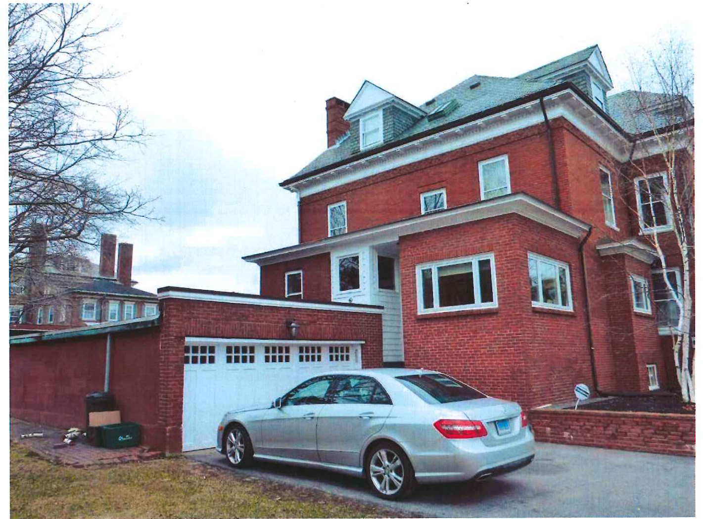
104 West Street. Detail of rear entrance.
