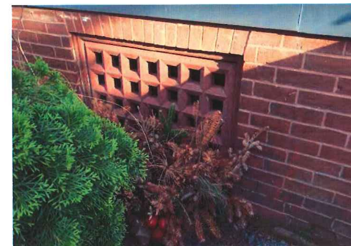
104 West Street. Lattice screen under front porch.
