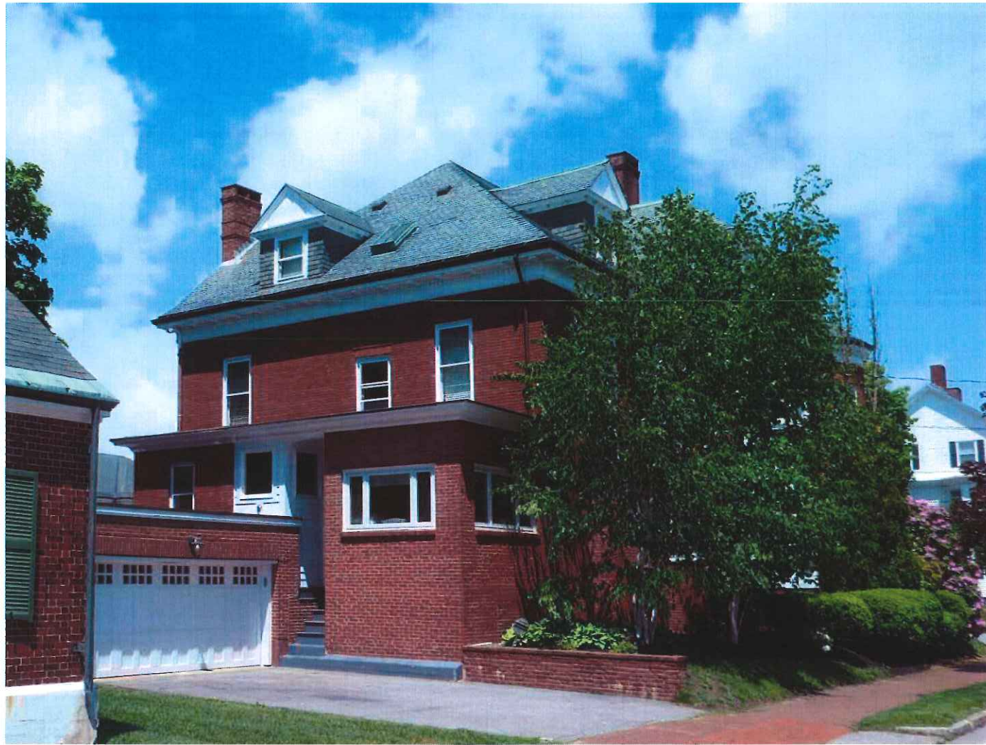
104 West Street. Current view from Chadwick Street.
