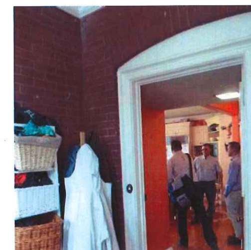
104 West Street. Original rear entrance doorway.
