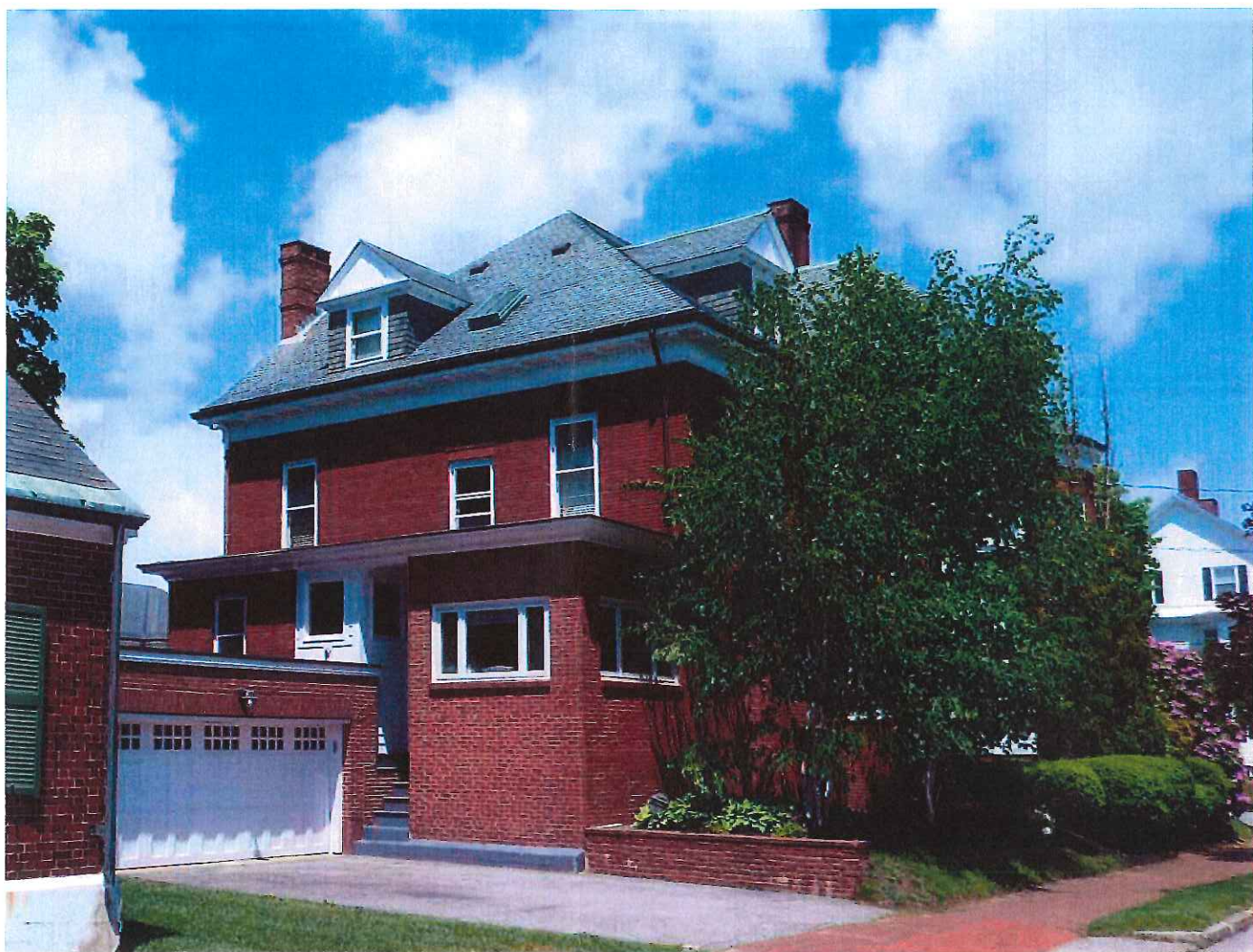
104 West Street. Current view from Chadwick Street.
