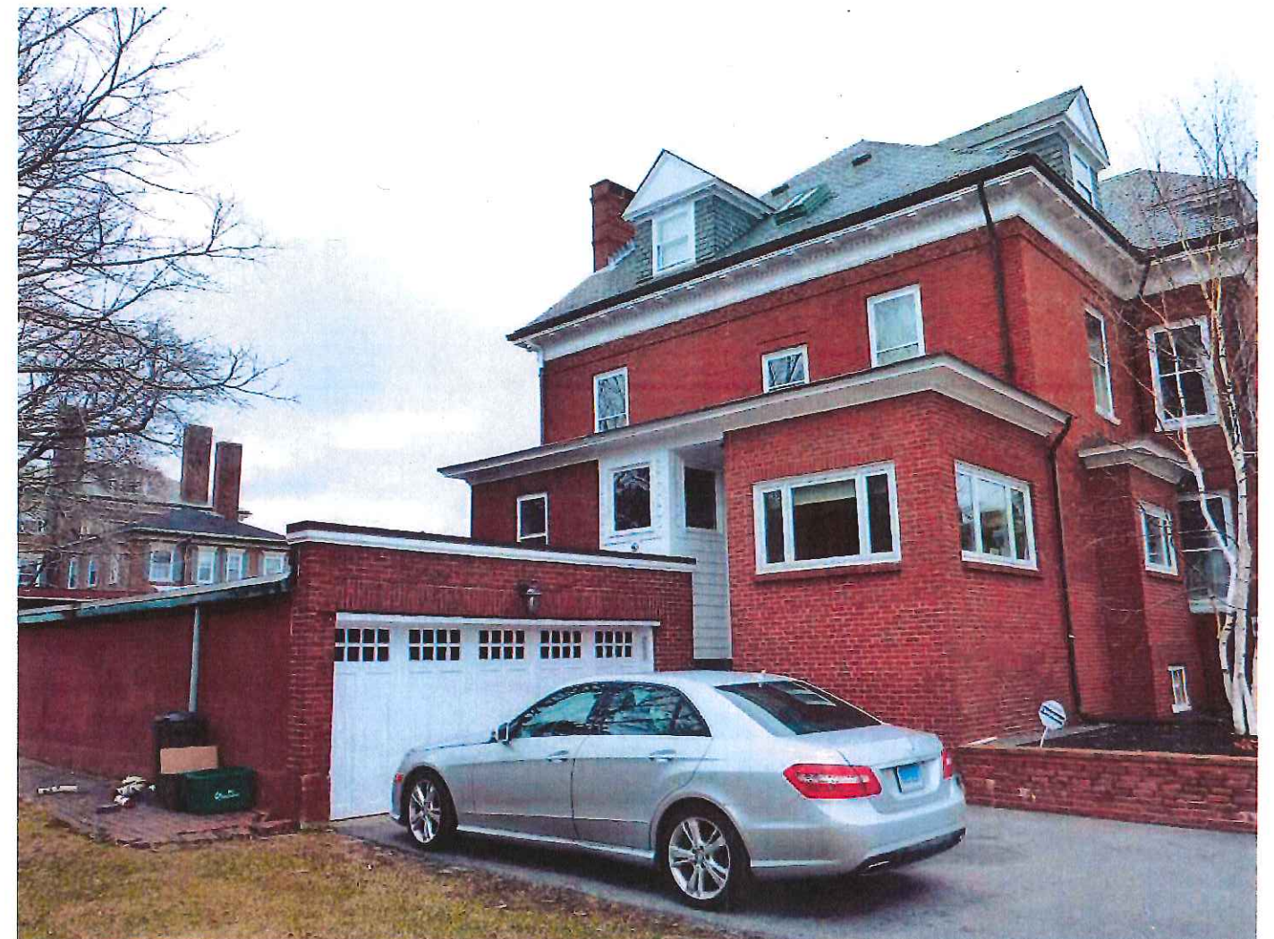
104 West Street. Detail of rear entrance.
