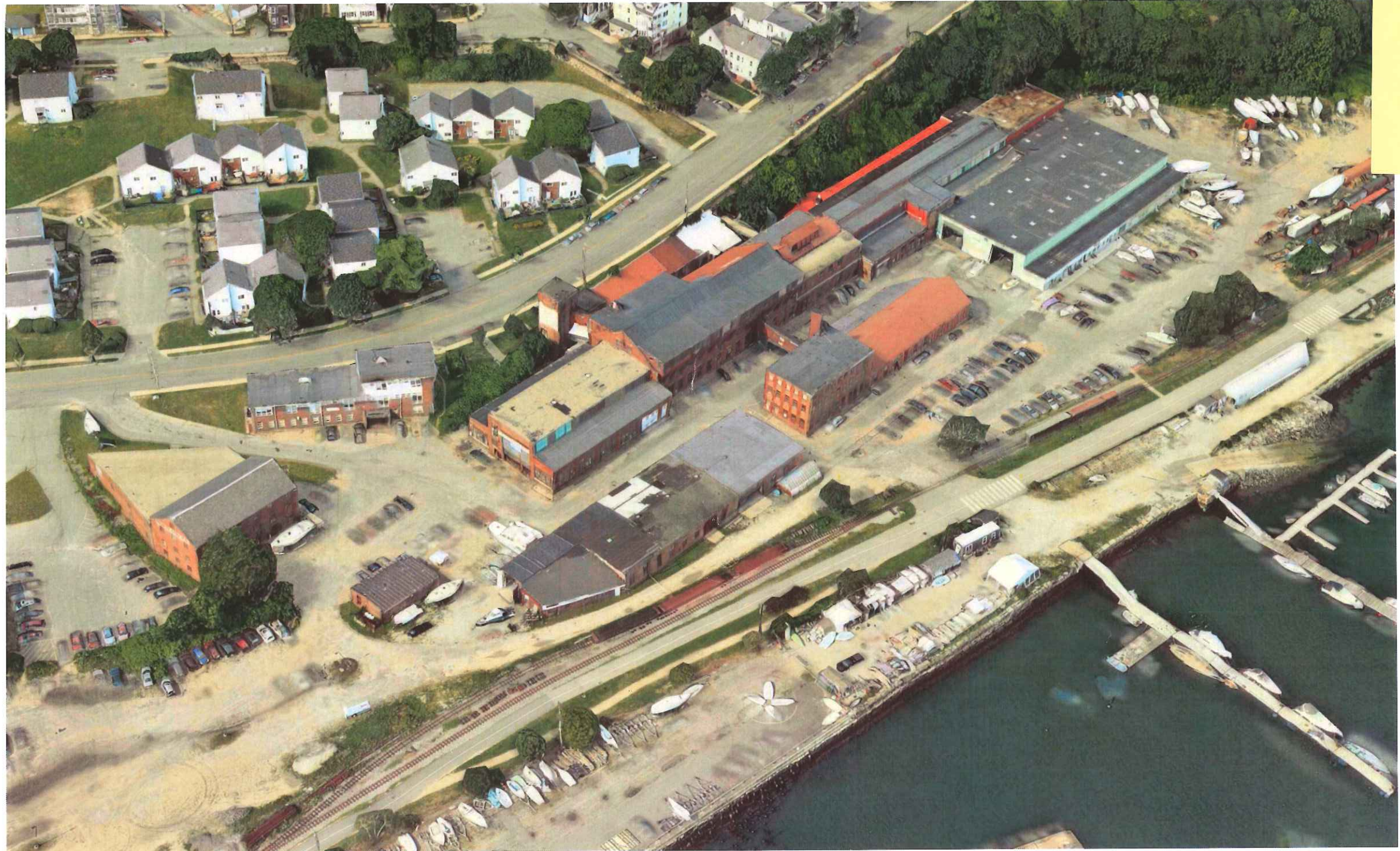
EXISTING AERIAL VIEW
