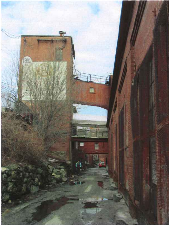
The pedestrian bridges connecting the manufacturing rows at the upper floor level are character-defining features of the industrial complex.
