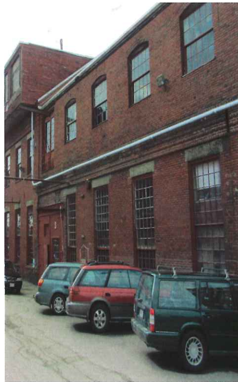
Windows within the manufacturing rows are typically large and multi-lite.
