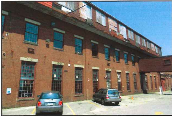
Building 2: Machine Shop Construction Date: c. 1847
