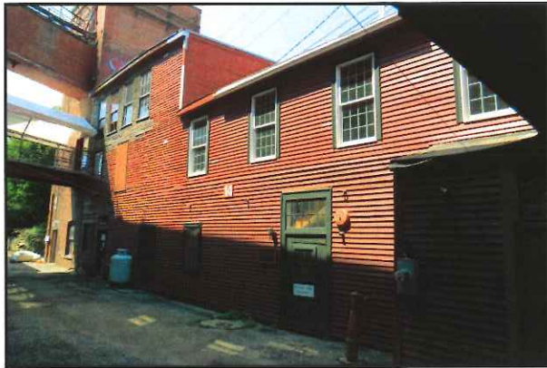
Building 14: Drafting Room and Storehouse Construction Date: 1858-64
