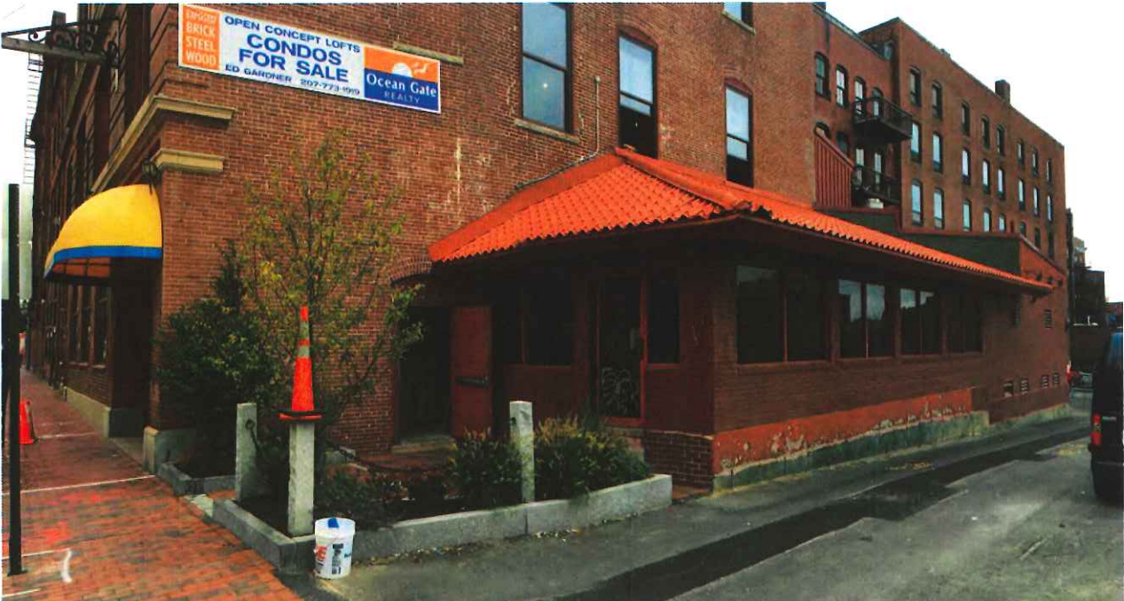
③ EXISTING CORNER VIEW
