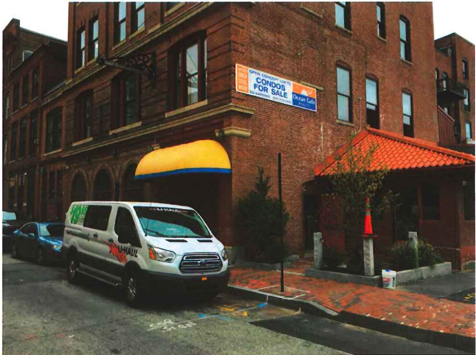
① Corner view
