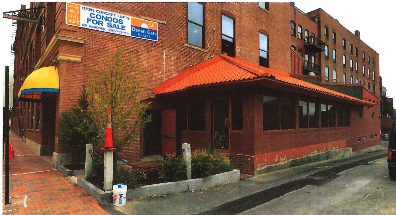
③ EXISTING CORNER VIEW
