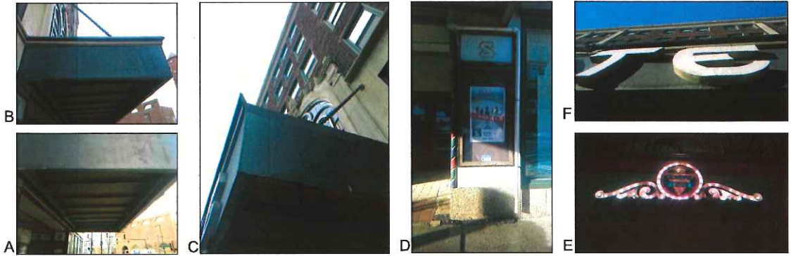
5 EXISTING CONDITION PHOTOGRAPHS SCALE: NTS
