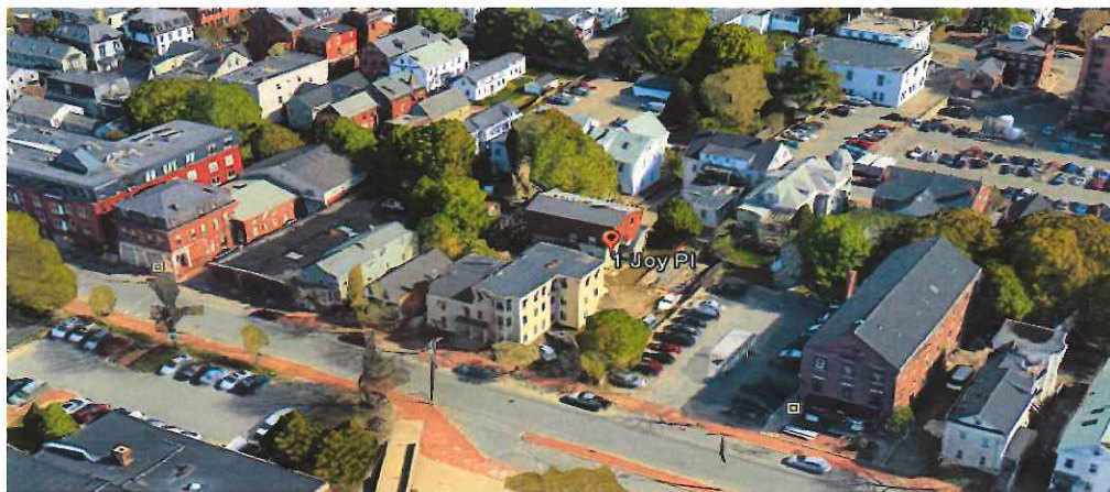
Access to Joy Place is from a private, shared-use road off of Brackett Street. Photo shows existing non-contributing structure at One Joy Place (red building). Large building in foreground (right side) is occupied by Fresh Approach Market.
