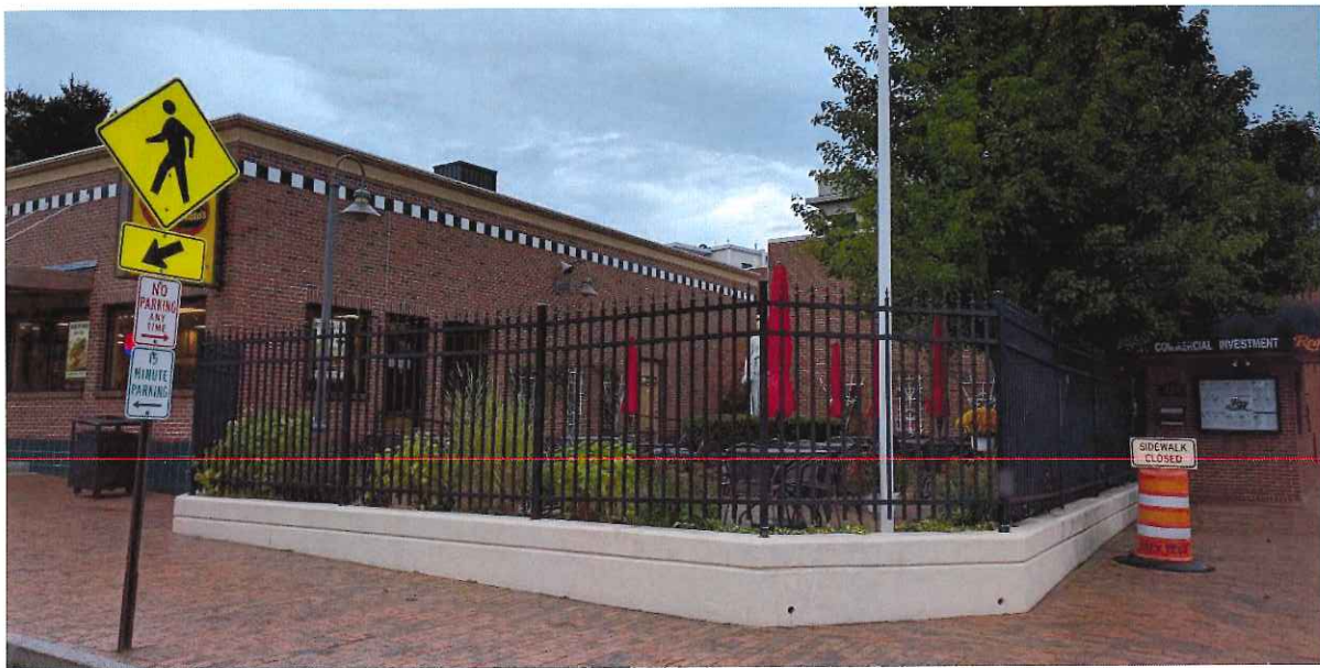
Close-up of existing foundation and dining garden.
