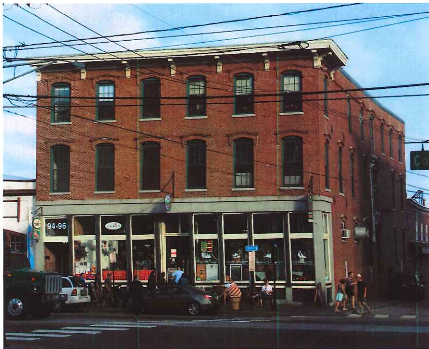
92-96 Commercial Street, existing conditions
