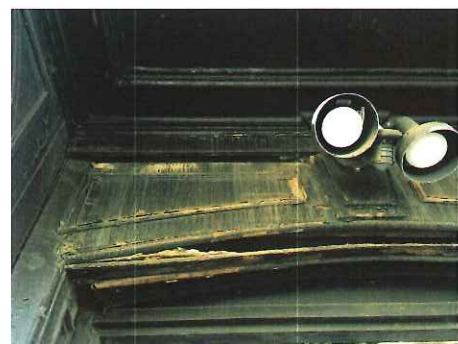
FIGURE G 126-128 Danforth Street Existing Wood Trim/Arch above glass transom
