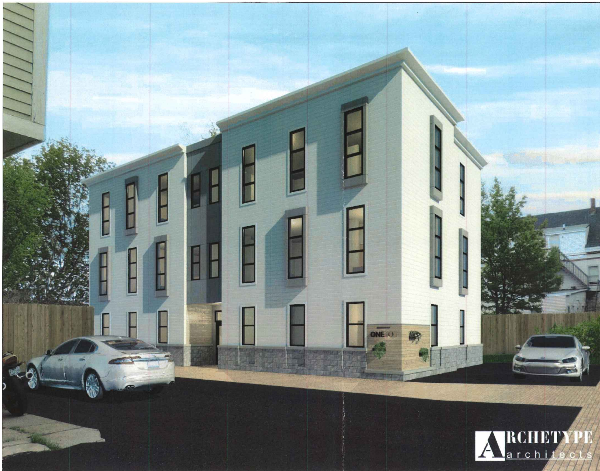
VIEW 4 - CLOSE UP ENTRY VIEW
