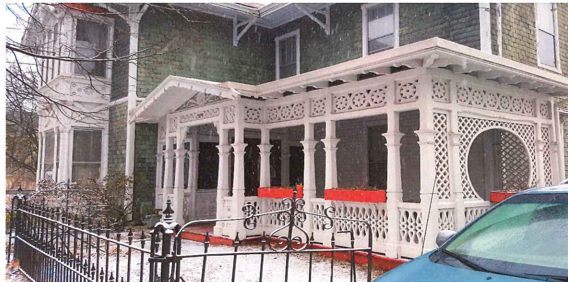
EXISTING HOUSE PORCH PHOTO
