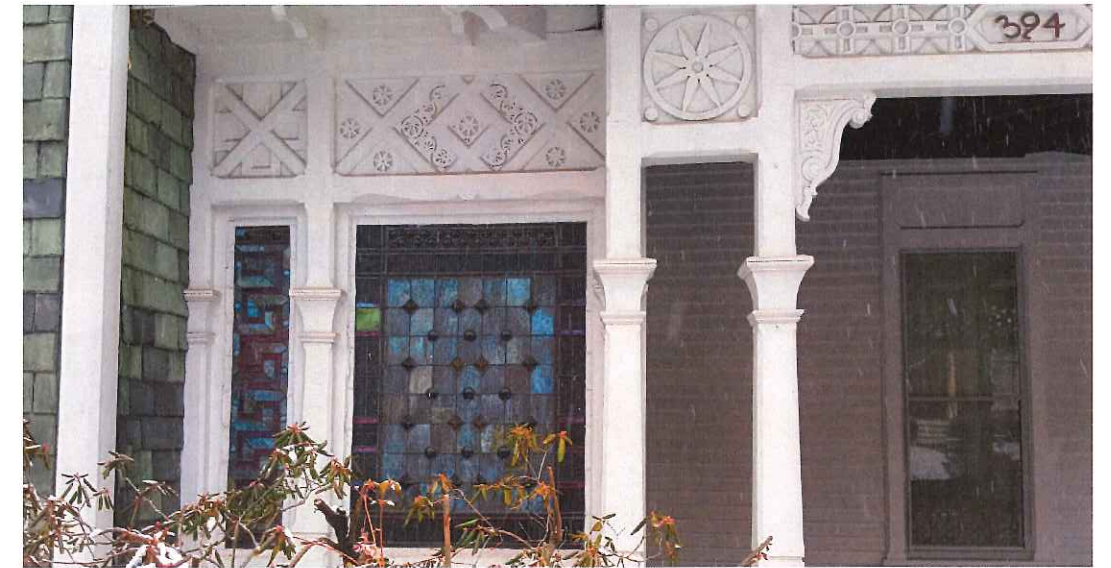
EXISTING ENTRY PHOTO
