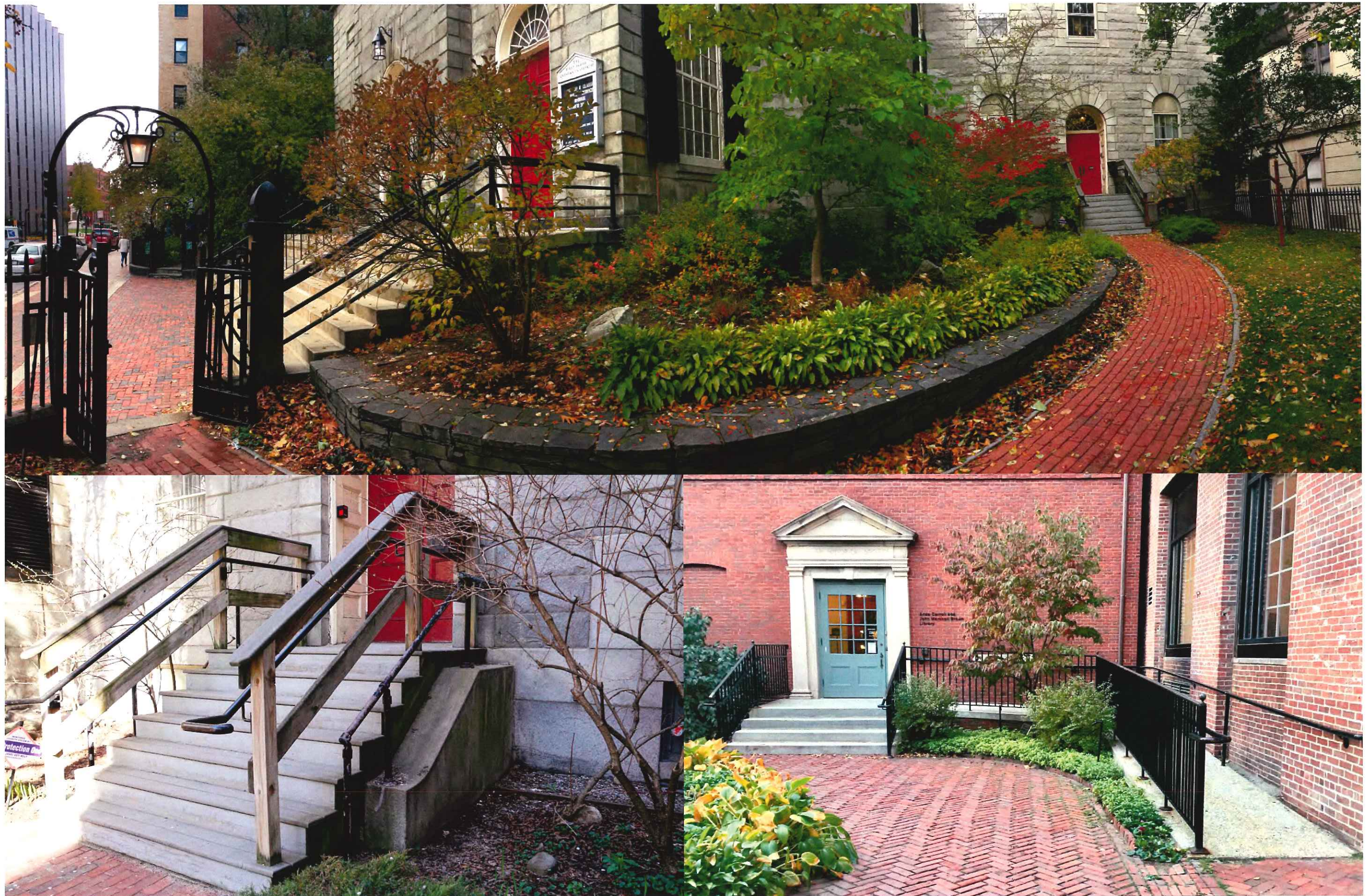
Top: Parish House Garden and Front entry stairs. Bottom Left: Original granite stairs with current overlay stairs, landing and handrails. Bottom Right: Maine Historical Society's painted steel guard and handrail system.
