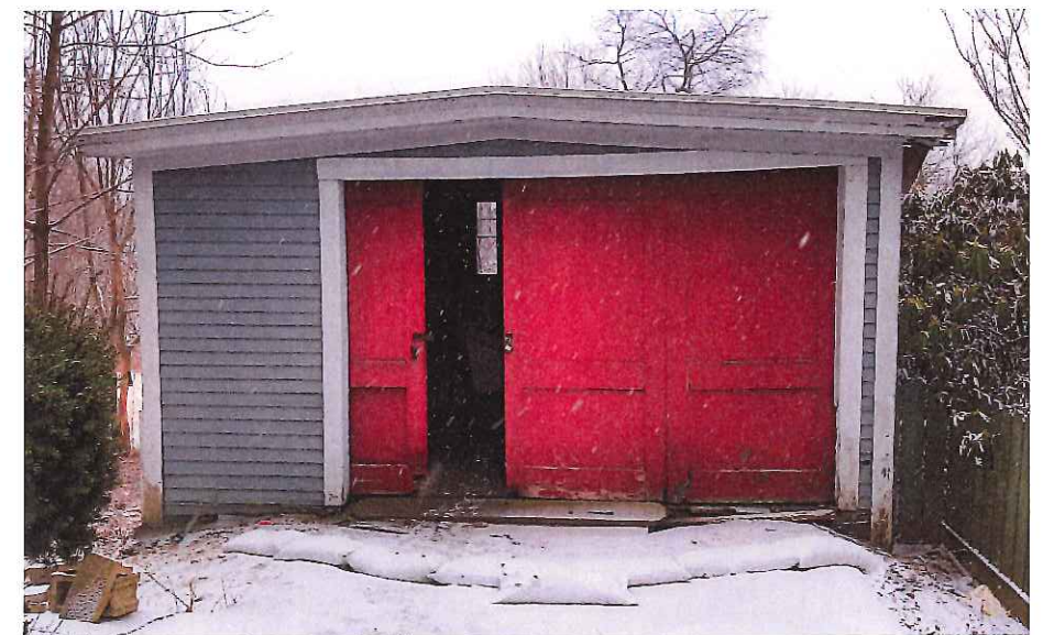
EXISTING GARAGE FRONT/NORTH PHOTO
