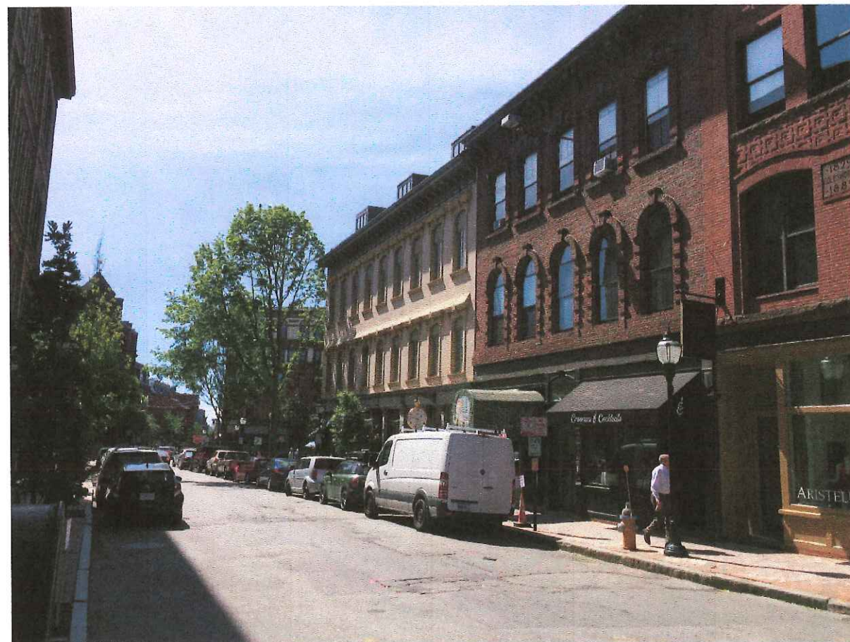
EXCHANGE STREET ELEVATION LOOKING TOWARDS TOMMY'S PARK
