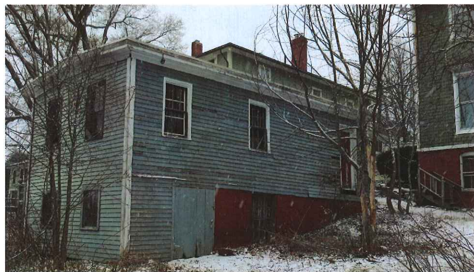
EXISTING GARAGE SOUTH EAST CORNER PHOTO
