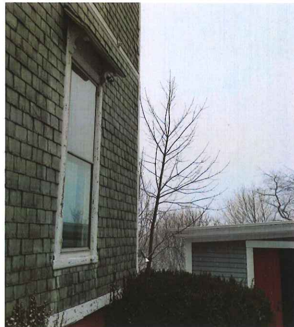
WINDOW TRIM ON HOUSE PHOTO
