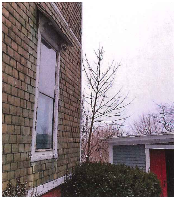
WINDOW TRIM ON HOUSE PHOTO
