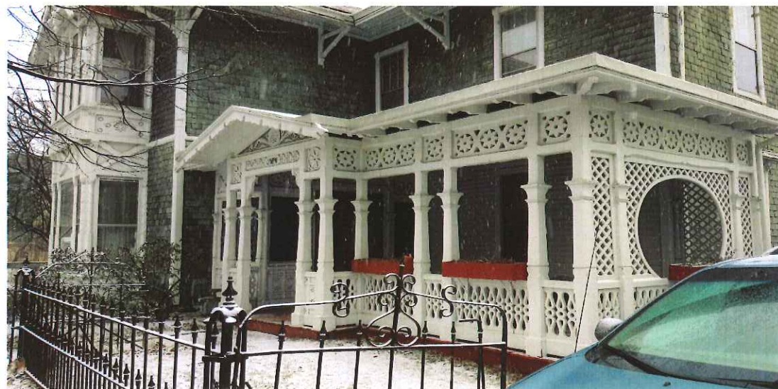
EXISTING HOUSE PORCH PHOTO
