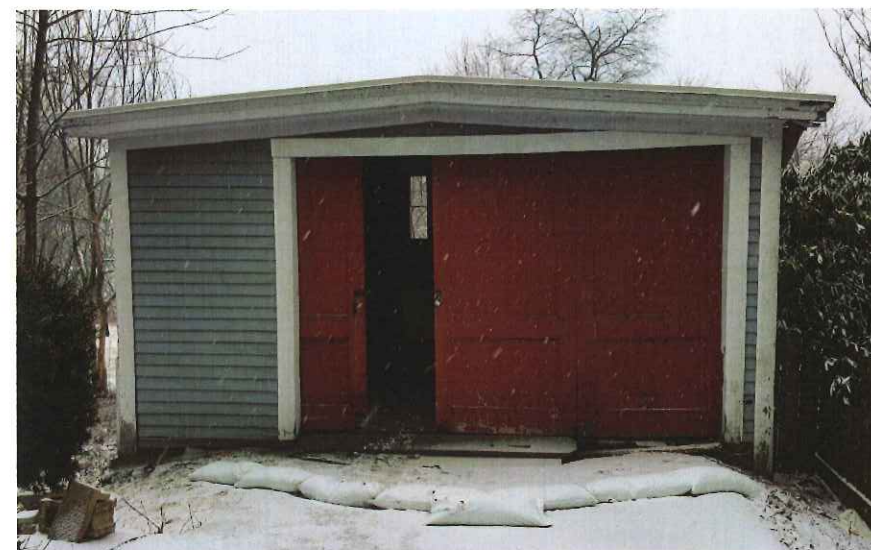
EXISTING GARAGE FRONT/NORTH PHOTO
