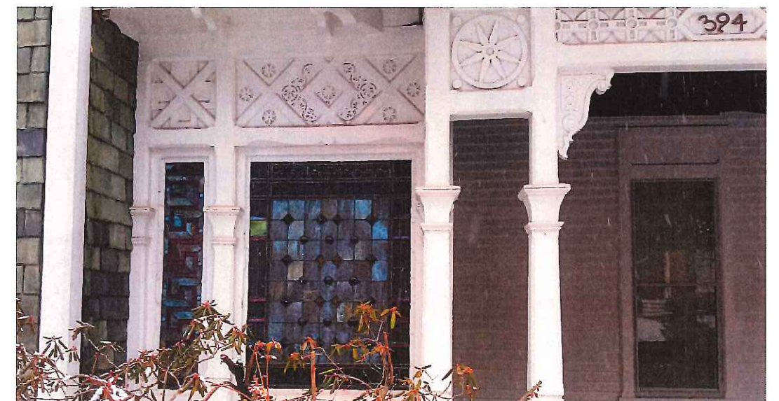
EXISTING ENTRY PHOTO
