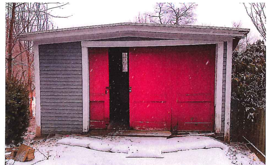
EXISTING GARAGE FRONT/NORTH PHOTO
