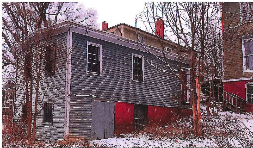
EXISTING GARAGE SOUTH EAST CORNER PHOTO
