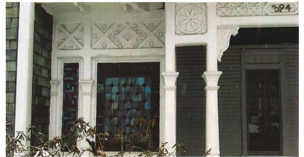
EXISTING ENTRY PHOTO
