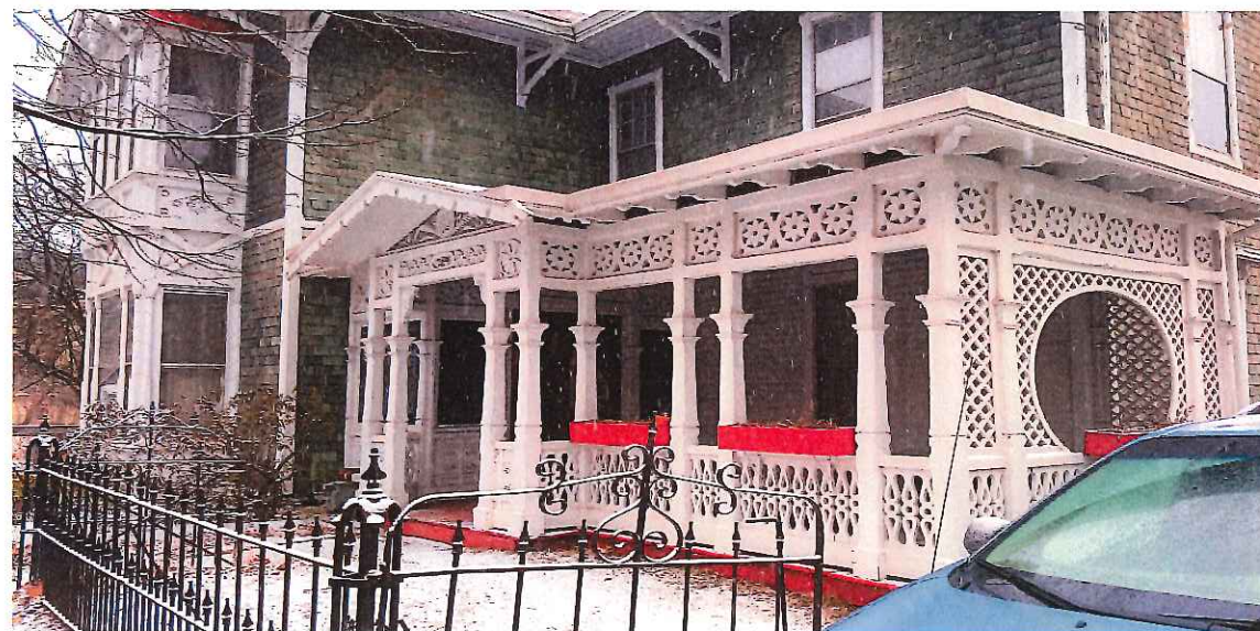
EXISTING HOUSE PORCH PHOTO
