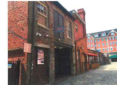
SITE CONTEXT (BUILDINGS WITH ADJACENT BLOCK ALONG WHARF STREET)
