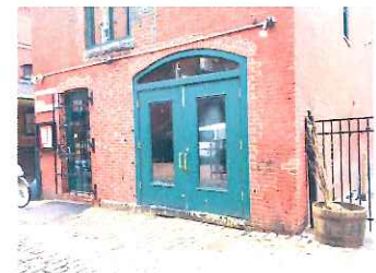
EXISTING FACADE PHOTOGRAPH (MAY 2017)
