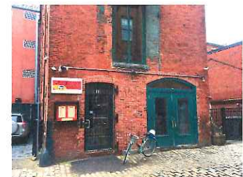
EXISTING FACADE PHOTOGRAPH (MAY 2017)
